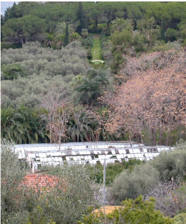
Fig. 2 – The abandoned park around the Costarainera sanatorium, seen from the cultivated property at its back: it is possible to recognize the central axis of the formal park, with exotic plants, and the patch of olive trees on terraces, on both sides of the upper part of the central main way.
